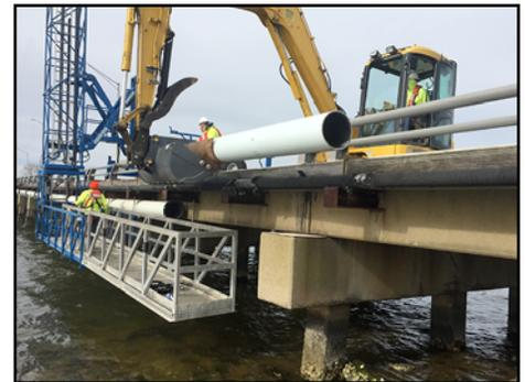
*Contractors replaced this section of the suspended pipeline in mid-February*
