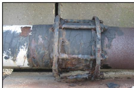
*The condition of the primary water pipeline to the fort made replacement necessary before work could begin on the secondary line.*
