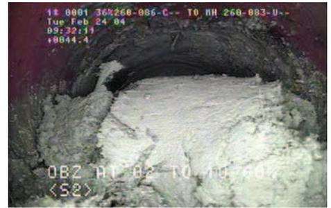
Just like melted butter, cooking grease eventually solidifies in the sewer system. The above picture is a Hampton Roads sewer pipe blocked by grease.
